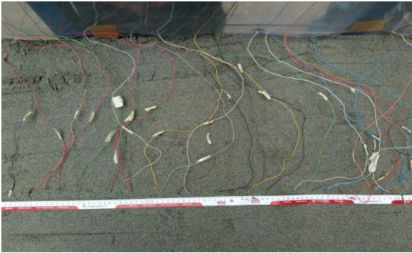
Fig. 2 – Miniaturized cables and electrodes deployed on the landslide body before being buried under 1cm of sand.
